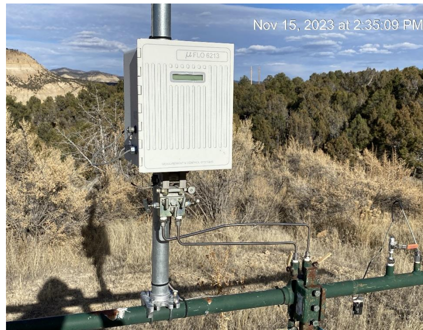
No visible display of gas meter calibration
