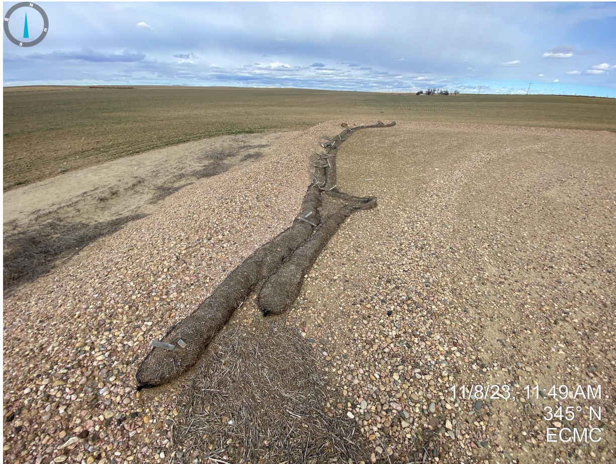
Photo 2. Degraded straw wattles observed on the northwestern portion of the location are now considered debris.
