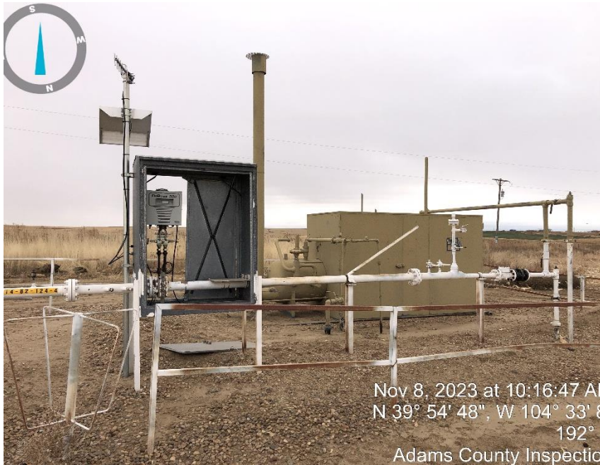
Photo #3 Meter & Separator.
