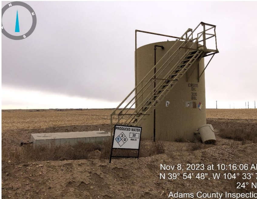
Photo #1 Crude tank & P/W vault.
