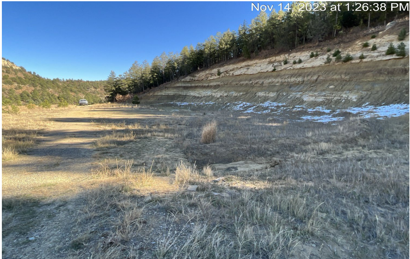
Photo 4. Facing southeast at the location. The location has not been recontoured and a steep cut slope remains. Previous corrective action not completed.
