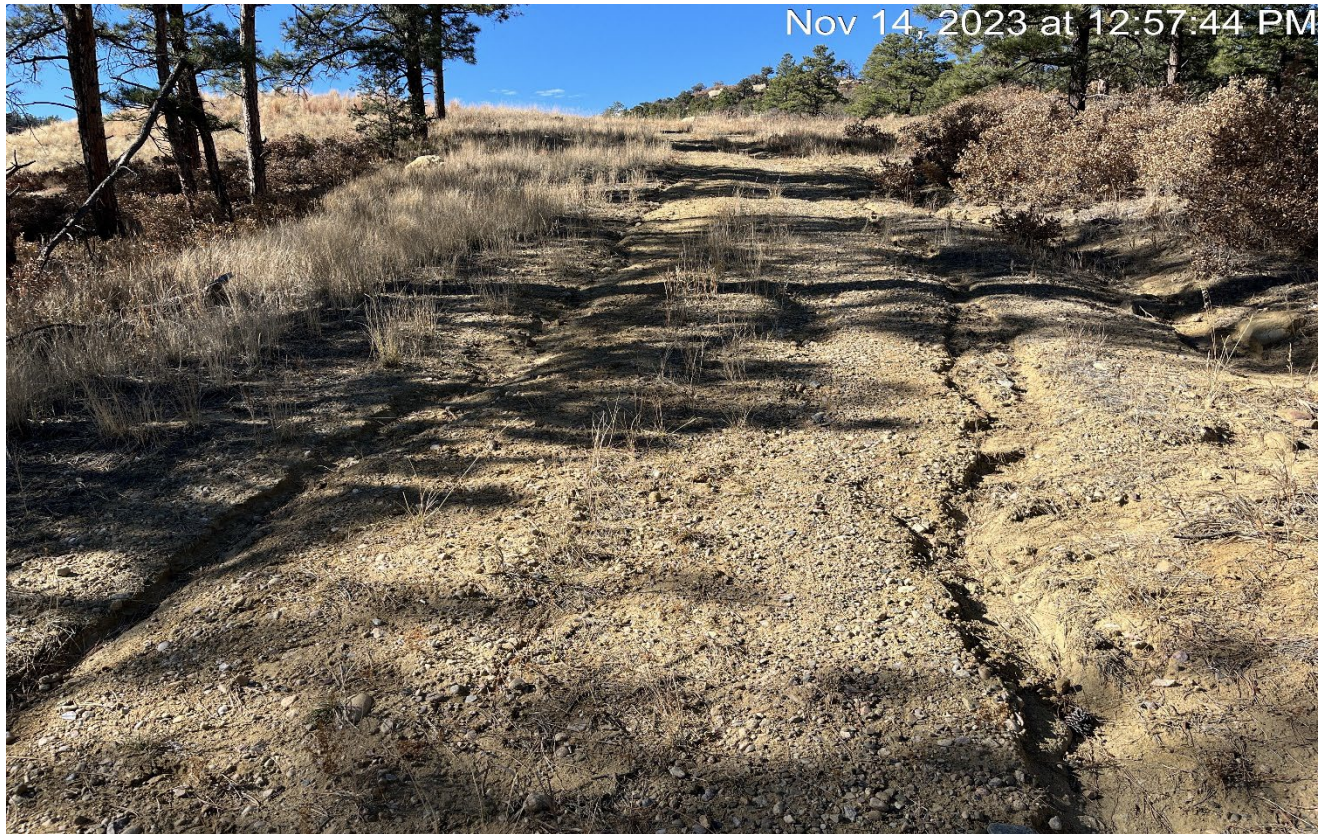
Photo 3. Facing northwest along the access road. There is erosion occurring along this area ascending to the location and will need to be repaired.
