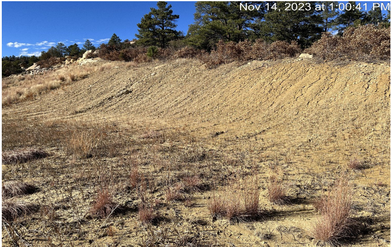
Photo 9. Facing northwest at the east cut slope. There is erosion along this area of the cut slope which is not yet stabilized.
