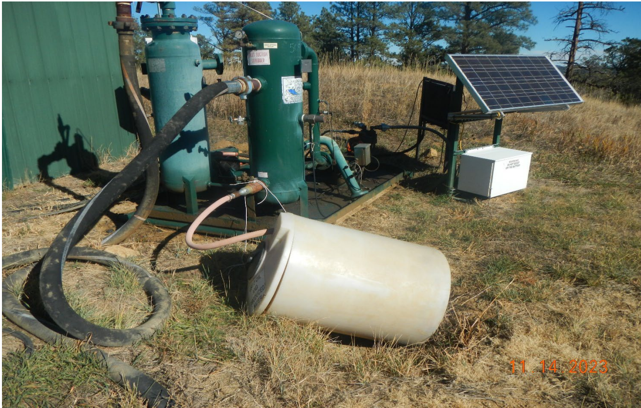
Photo 4. This container has fallen over and needs to be installed with containment..
