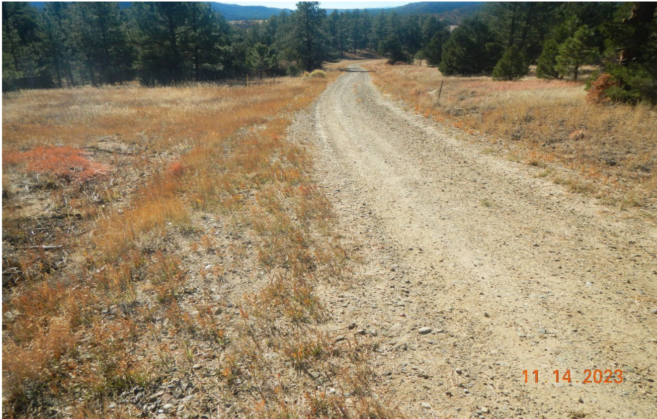
Photo 1. Facing southwest along the access road which is stabilized with BMP's.
