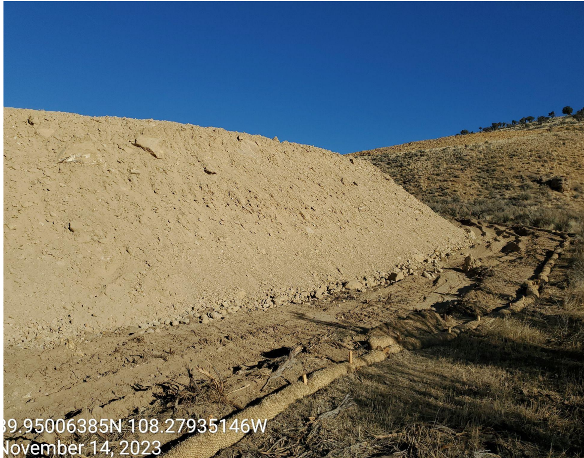
Photo 4: Photo example of slopes along the Location that will require additional stabilization control measures. Soils at risk to wind and water erosion; fugitive dust control measures required.
