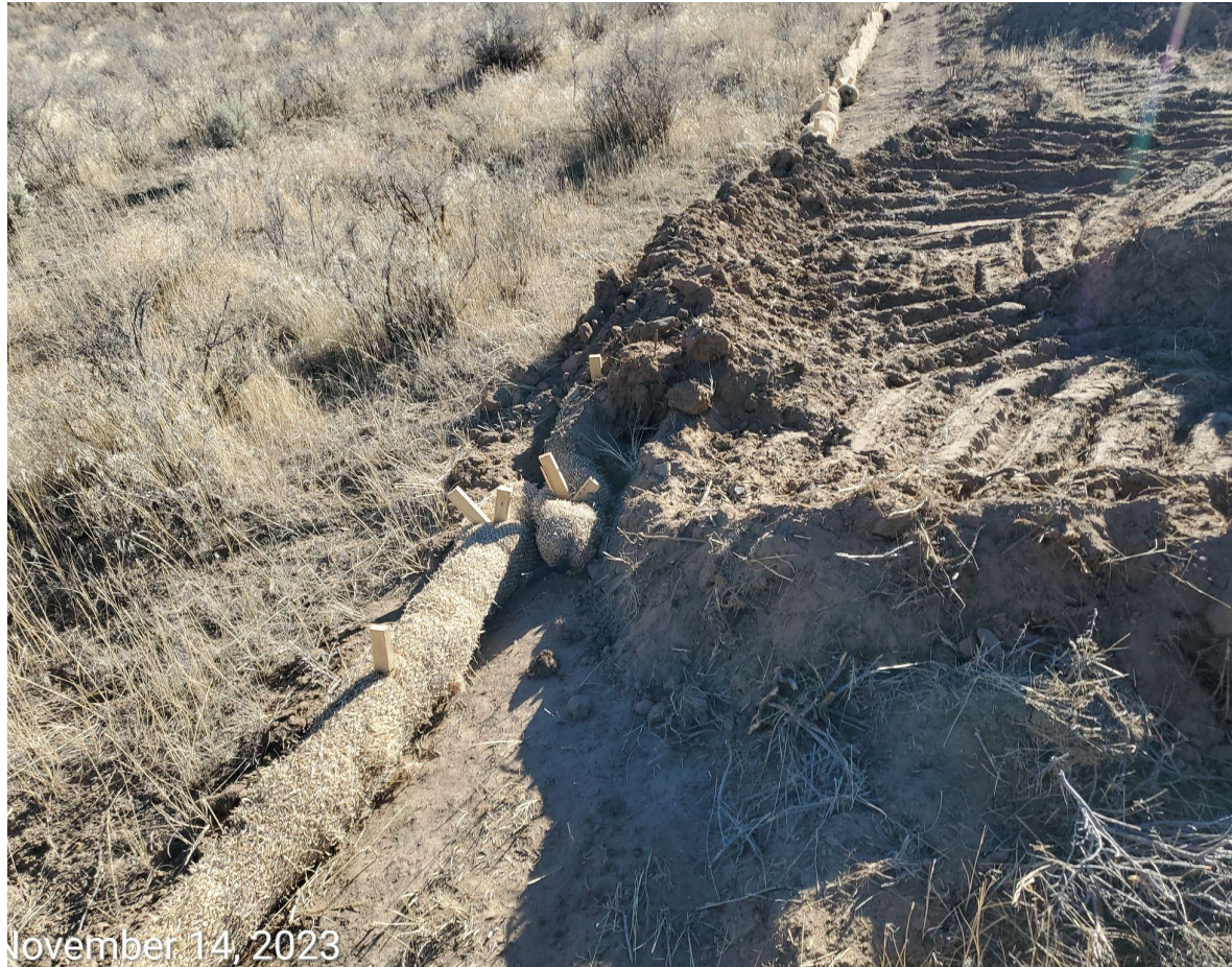
Photo 3: Photo example showing area where soils have been pushed over the erosion logs during construction.
