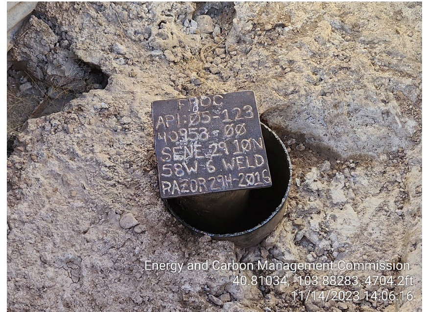
Photo 6 – Razor 29H-2016 – PA'd – Cut and Capped
