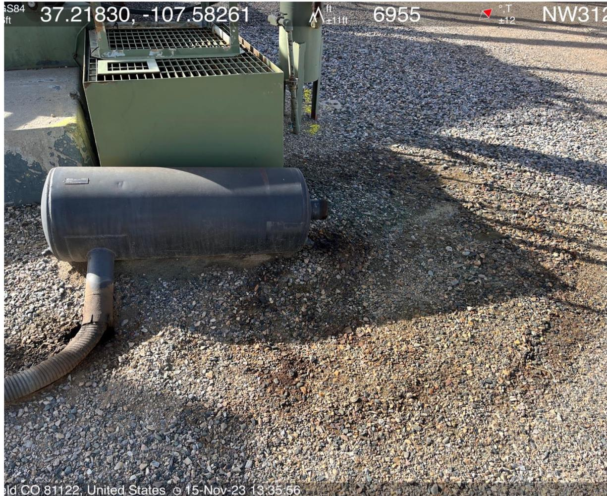
Photo #9 View of impacted material on ground at muffler.
