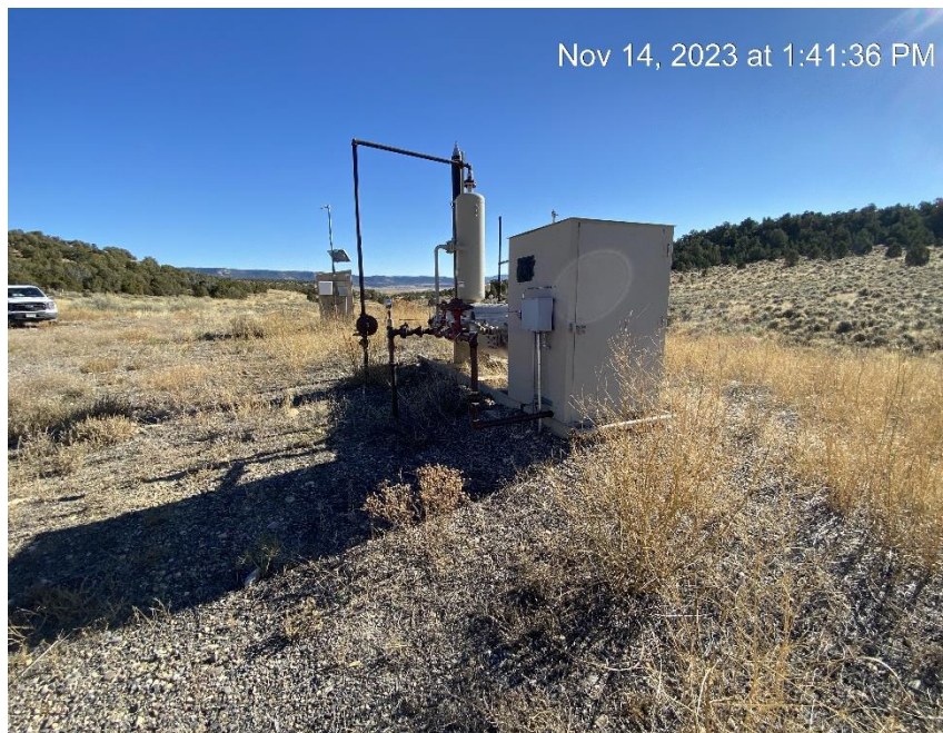
Separator and gas meter run
