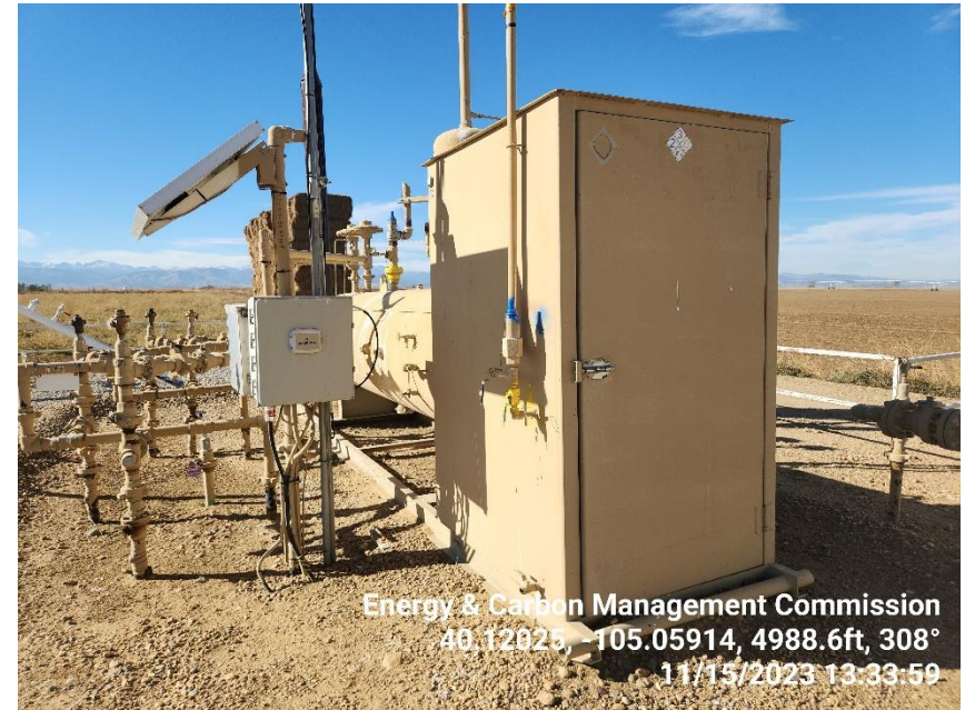
Photo 5 Horizontal Heated Separator.
