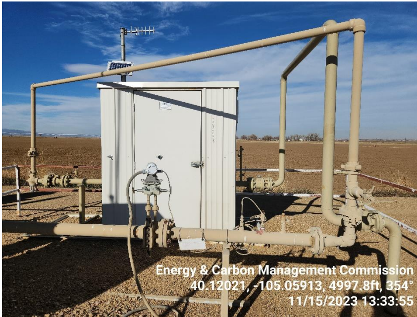
Photo 5 Gas Meter Run.
