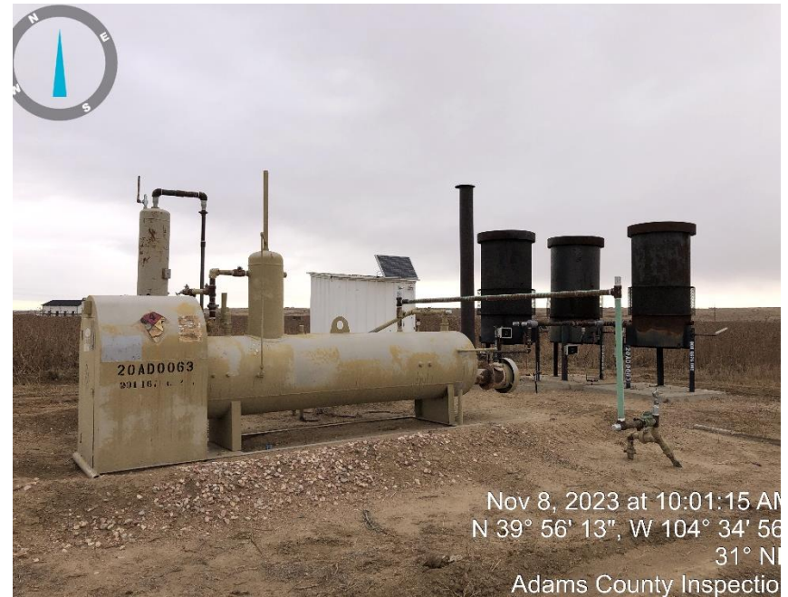
Photo #4 Separator, Meter house & EDCs.
