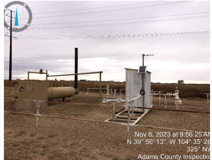
Photo #4 Separator & meter house.
