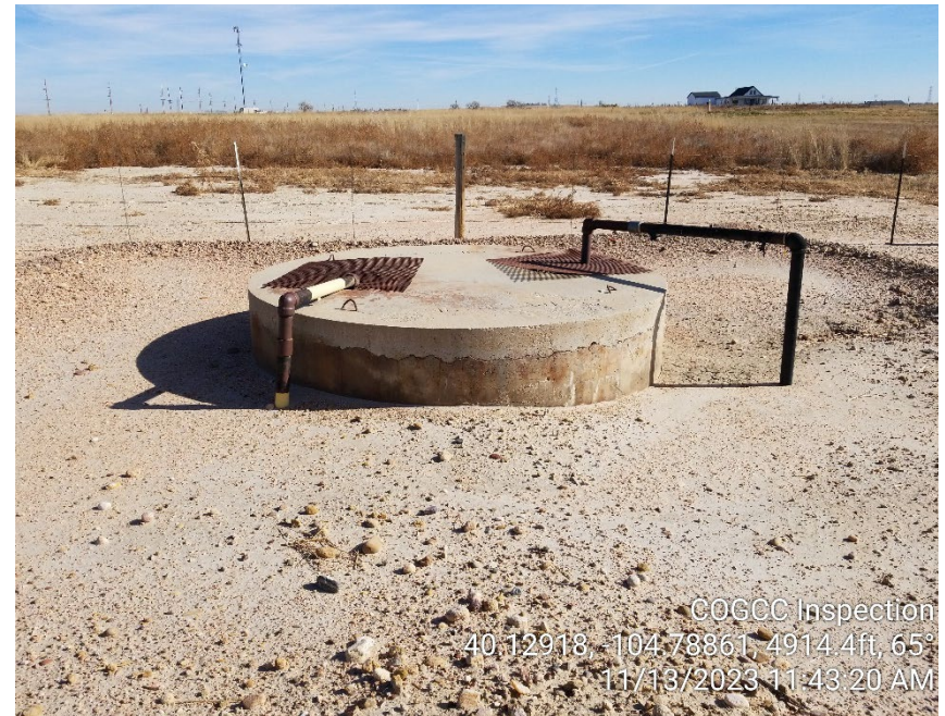
Photo 6 - Produced water vault.
