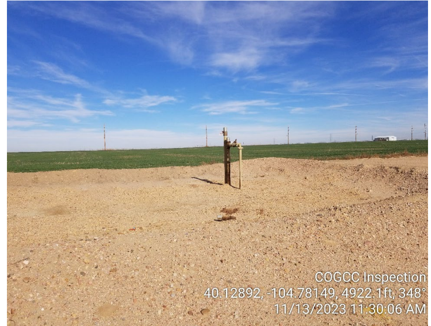
Photo 2 - Former tank location. Impacted soil visible.
