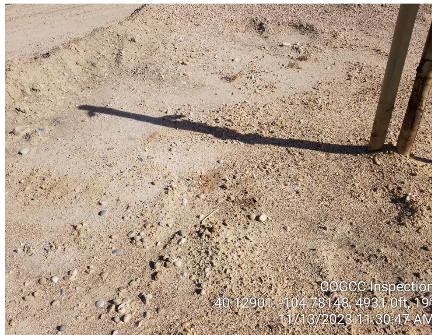
Photo 4 - Former tank location. Impacted soil visible.
