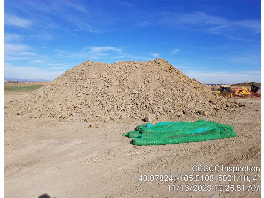
Photo 2 - Backfill dirt stockpile. Backfill in process – AM inspection.
