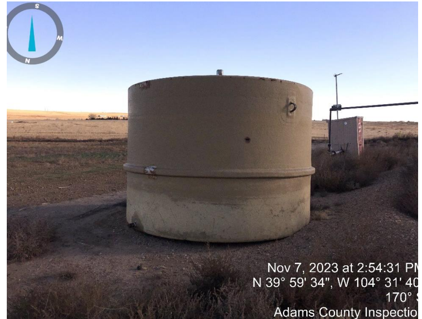
Photo #4 Produced water tank out side containment and not connected.
