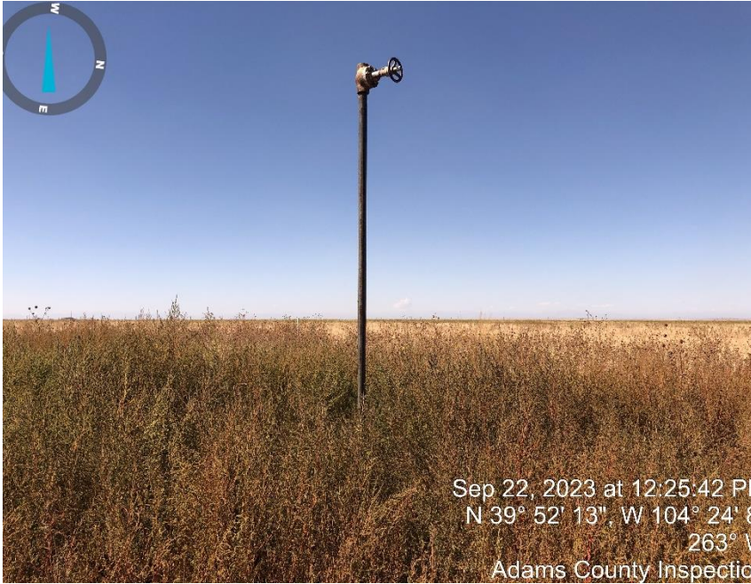
Photo #1 Well head.
