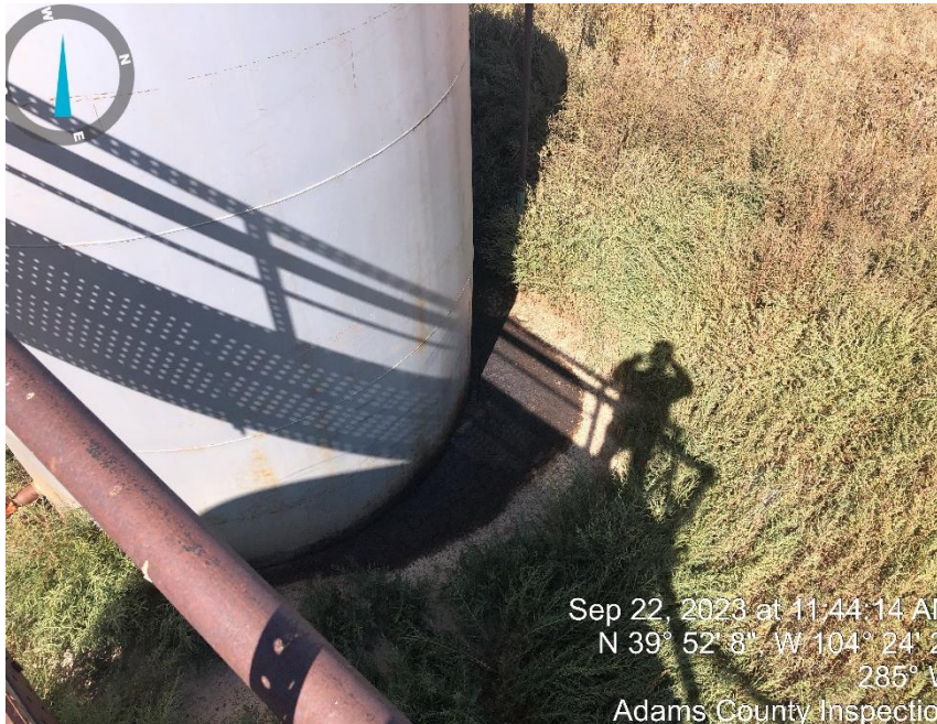
Photo #3 Stained soil around crude tank in containment.
