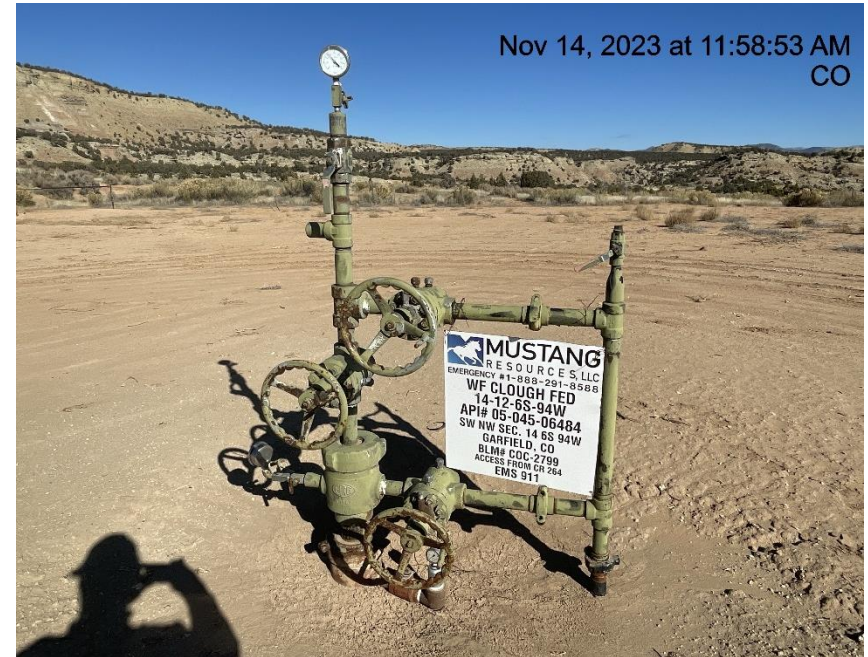
Photo # 6598 Meter calibration info not conspicuously posted, no meter on location & no signage as to where meter is located.
