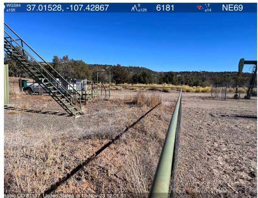
Photo #2. Corrective action not completed.
