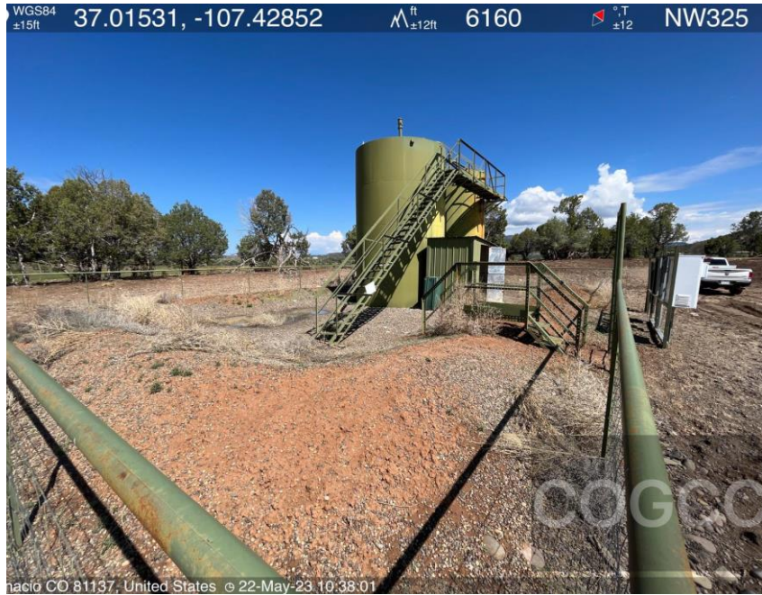
Photo #1. Corrective action identified in FIR Doc.#712700199.
