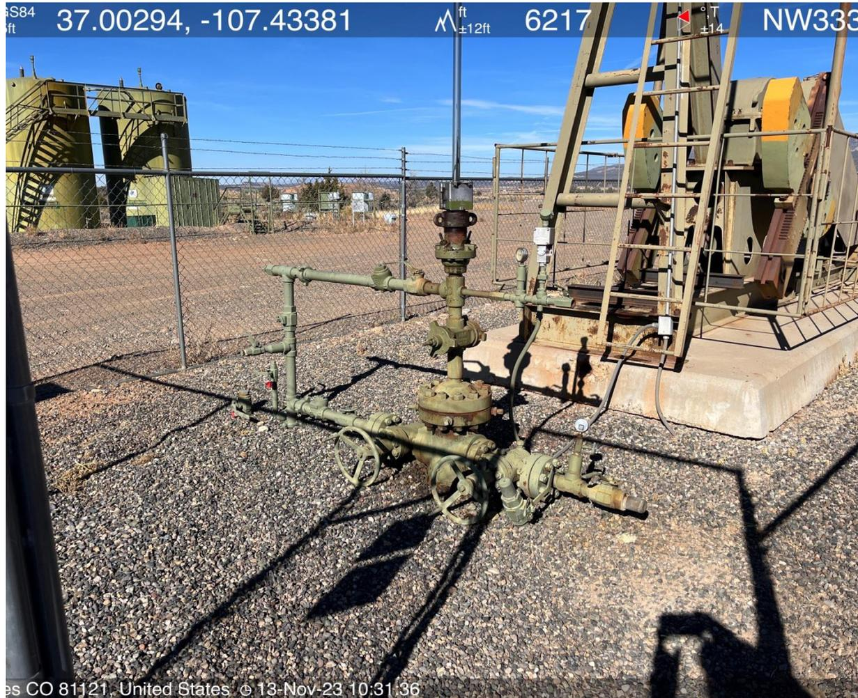
Photo #2 View of the Gallegos 9-2 wellhead assembly.
