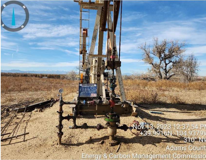
Photo 1 well head and equipment
