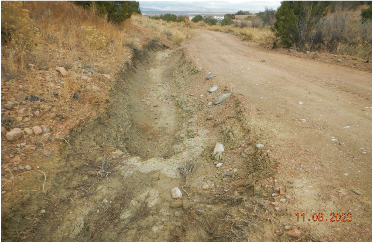
Photo 1. Facing north along the access road. A recent storm event has created an erosion gully along the roadside which needs to be repaired.
