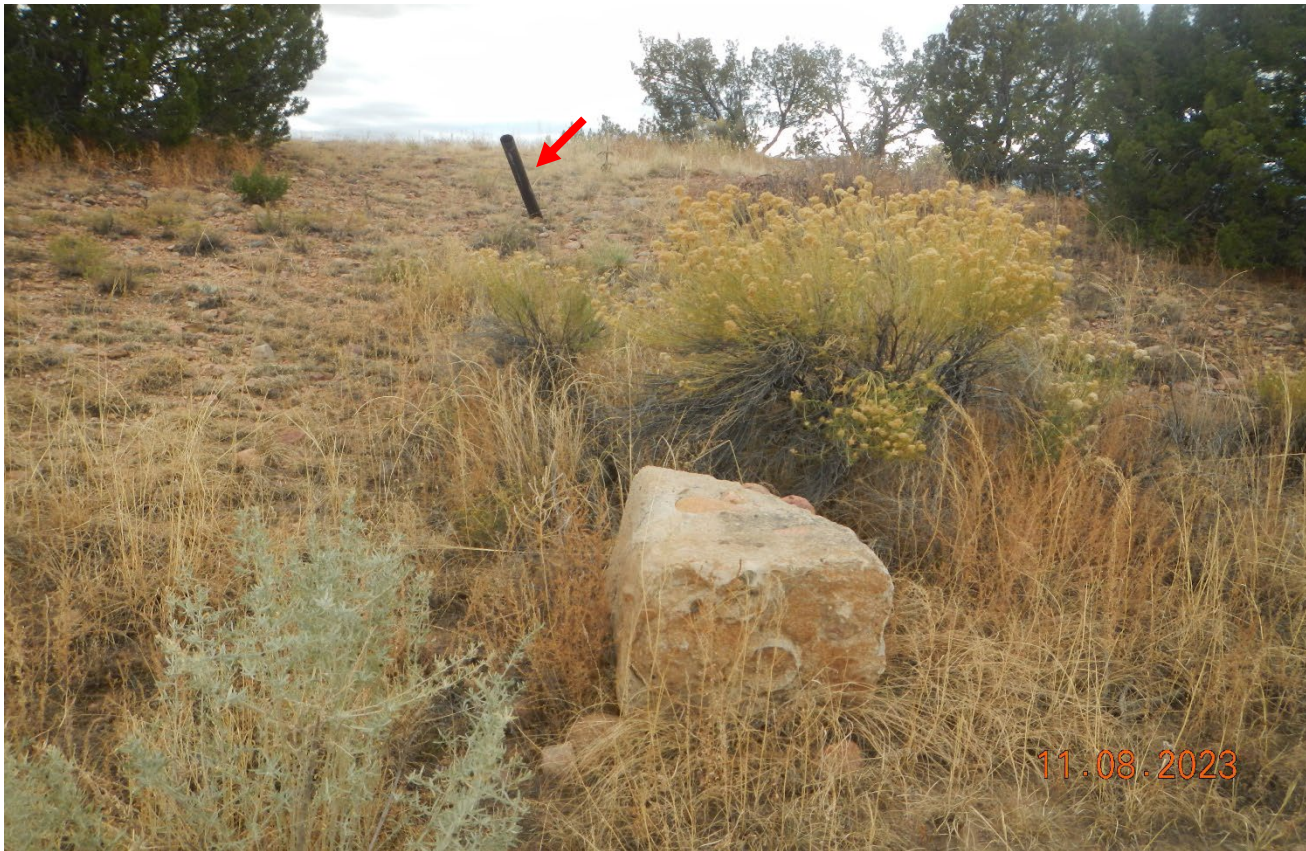
Photo 5. There is a cement block and guy line anchor that remains at the east side of the location that needs to be removed.
