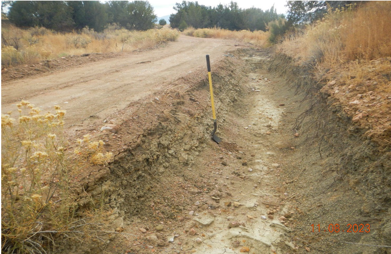
Photo 2. Facing back south toward the erosion gully along the roadside which needs to be repaired. A 4.5 ft. shovel shows depth of erosion.
