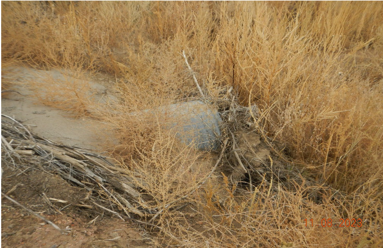
Photo 3. The culvert at this drainage crossing has filled in with sediment and debris and must be cleaned out.
