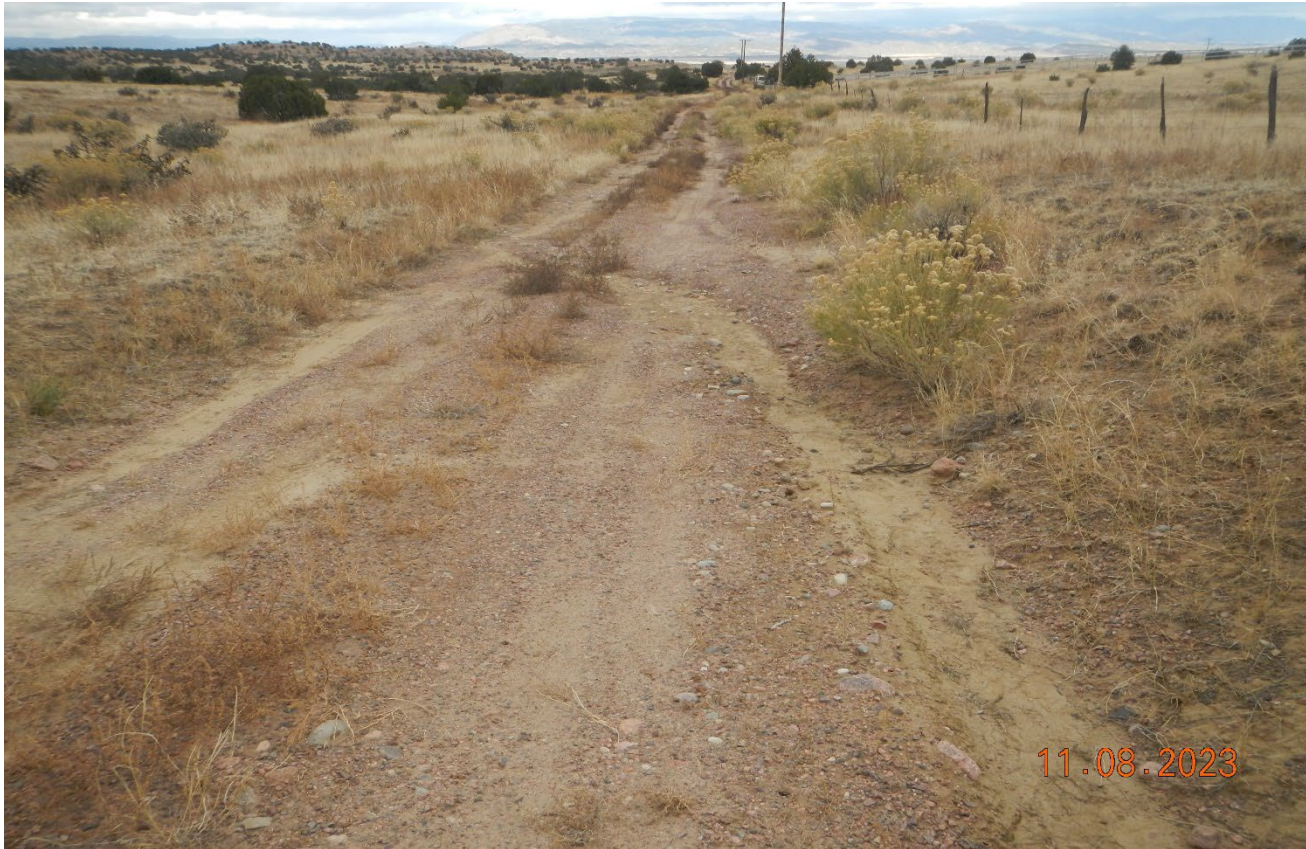
Photo 1. Facing north along the former access road. There is erosion along the road that must be repaired.
