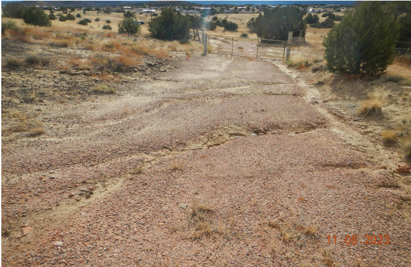
Photo 2. Facing southwest toward the access road which must be reclaimed. There is erosion occurring along this area that needs to be repaired and stabilized.
