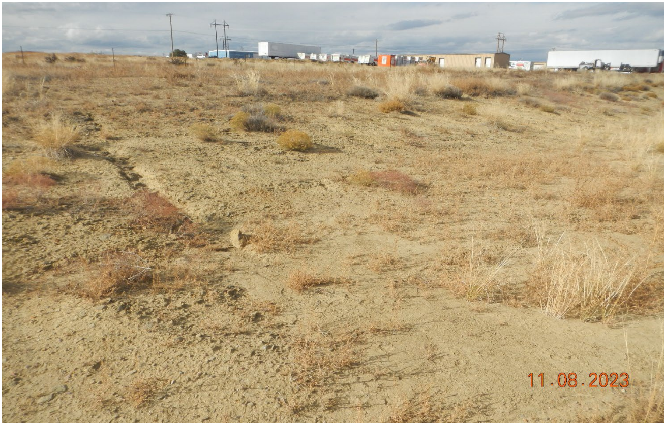
Photo 6. Facing northwest along the cut slope. There is rilling erosion along the cut slope which is not stabilized. Previous corrective action was not completed.
