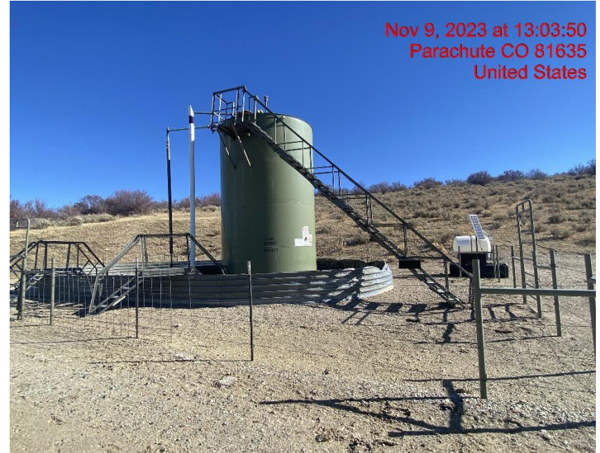
Tank Battery – Photo #07455
