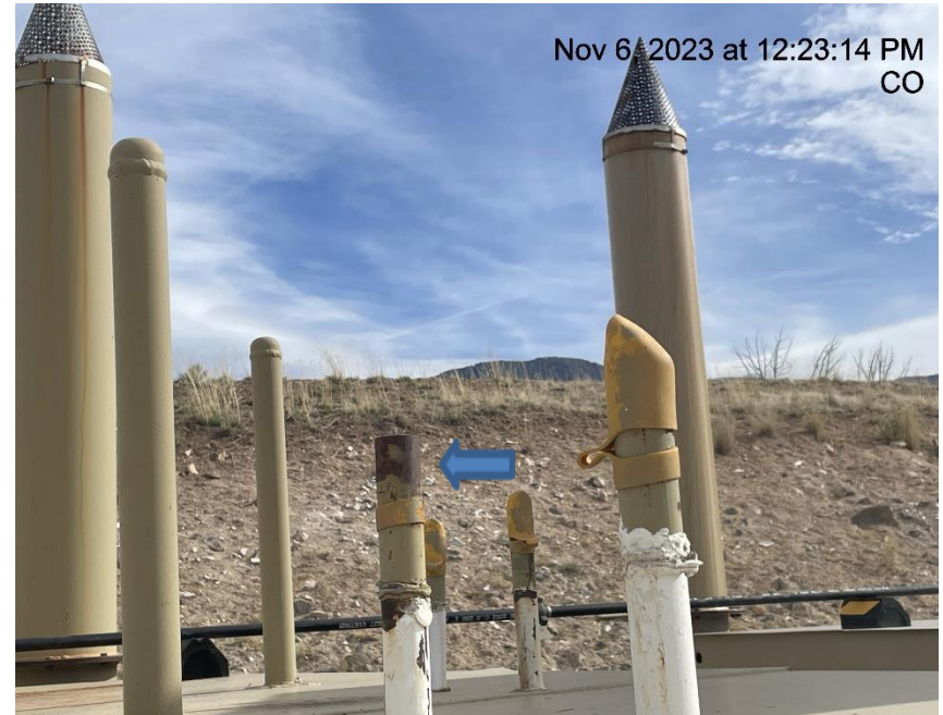
Photo # 5603 PRV vent line lacks cap
