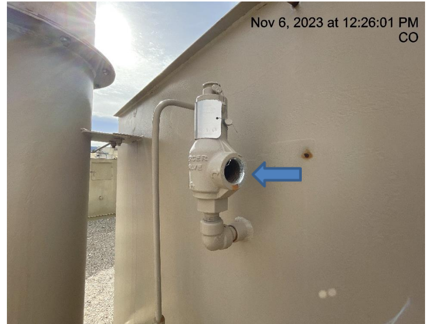
Photo # 5599 PRV lacks vent line
