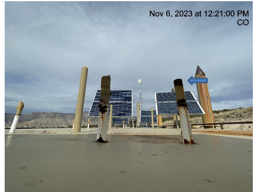
Photo # 5601 PRV vent line lacks cap
