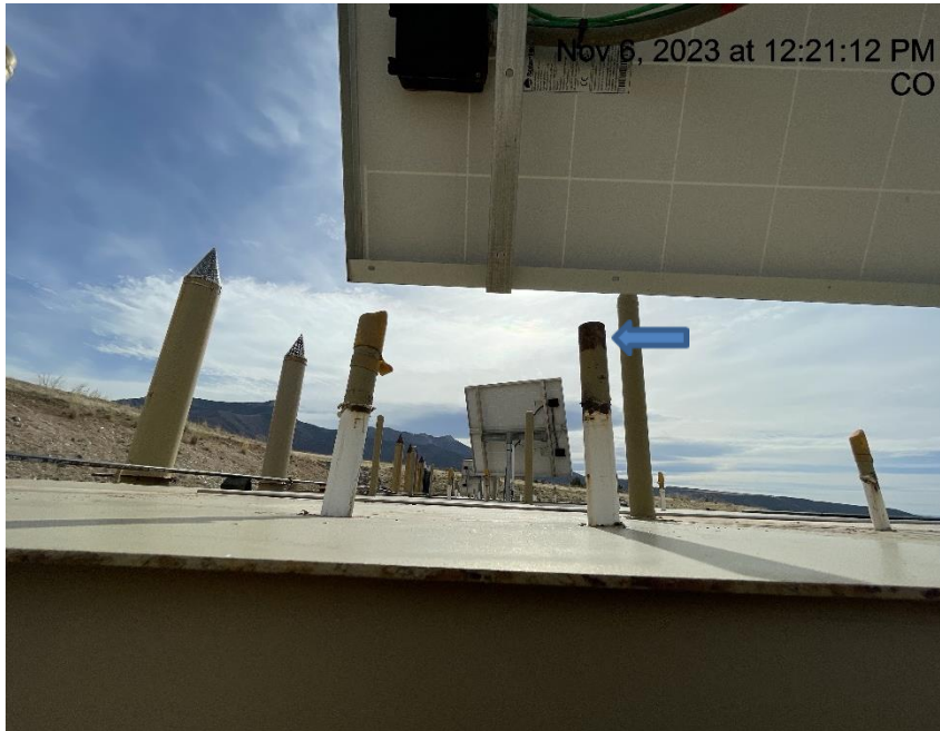
Photo # 5602 Rupture disc vent line lacks cap
