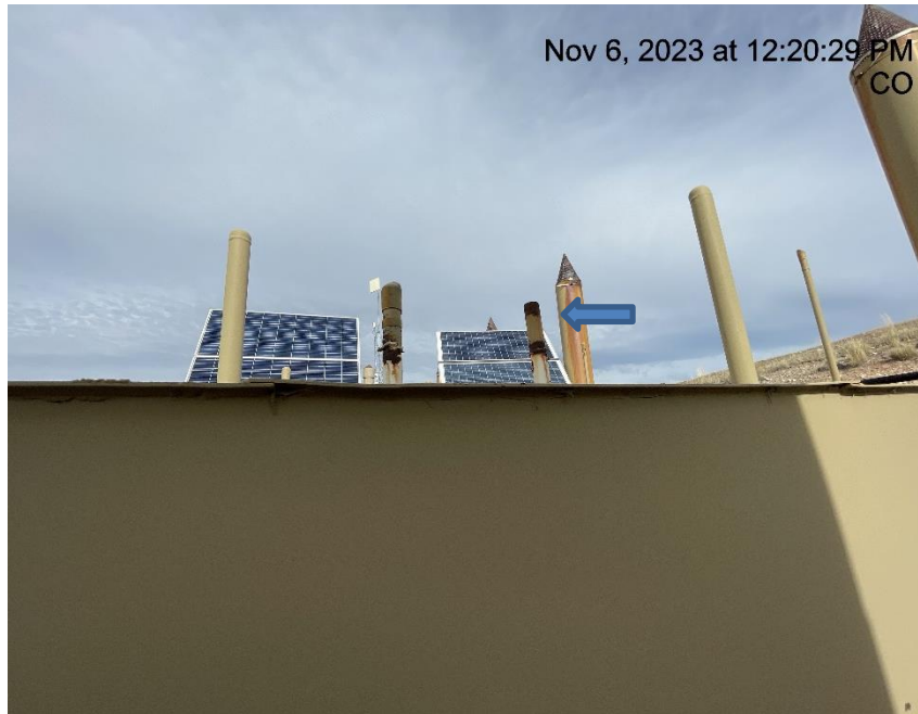
Photo # 5600 PRV vent line lacks cap
