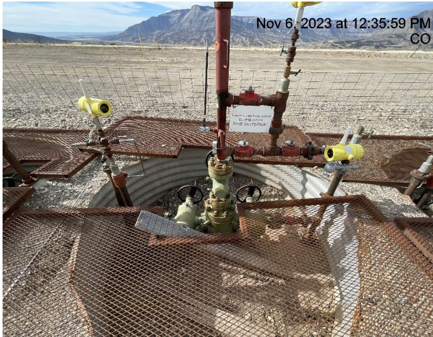
Photo # 5596 Multiple cellar covers improperly placed & only partially covering wellhead cellars
