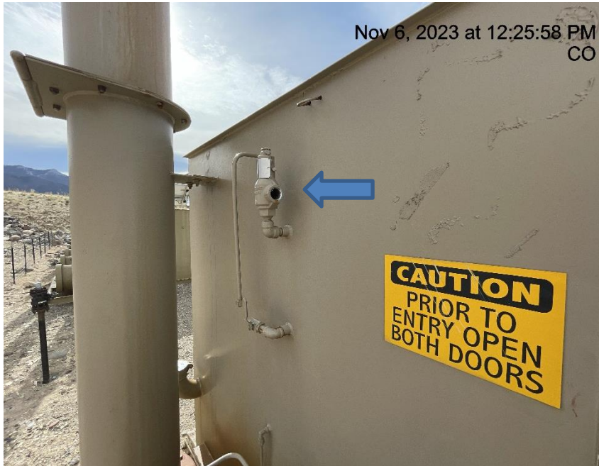
Photo # 5598 PRV lacks vent line
