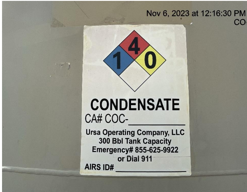
Photo # 5594 Tank label contains inaccurate information
