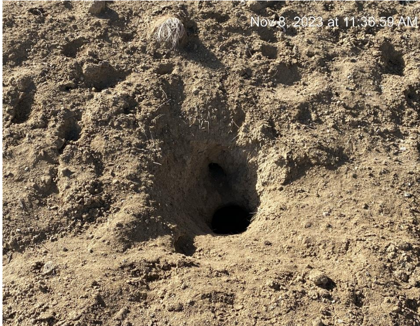
Tank berm burrows
