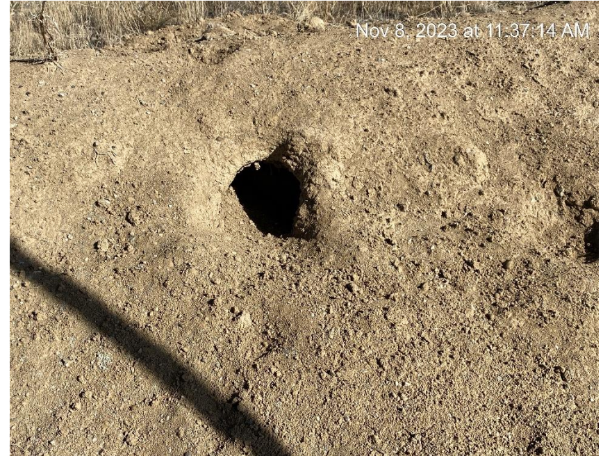
Tank berm burrows
