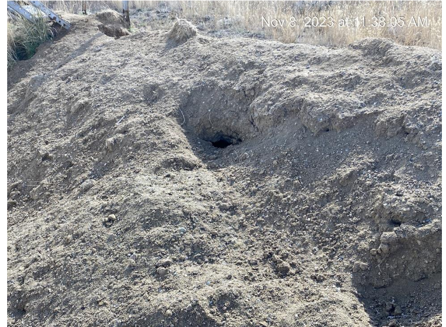
Tank berm burrows
