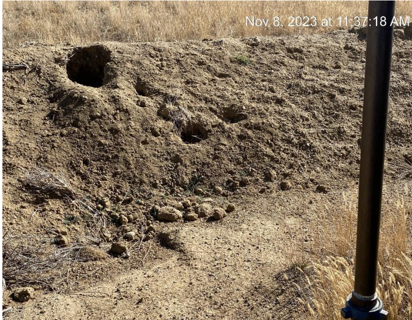
Tank berm burrows
