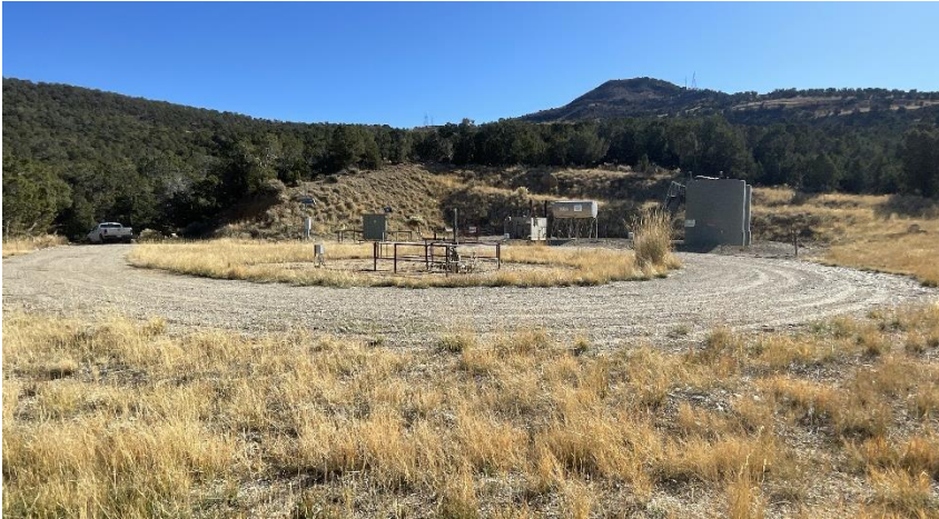
North West corner of location.
