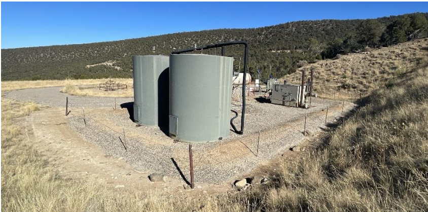
South West corner of location.
