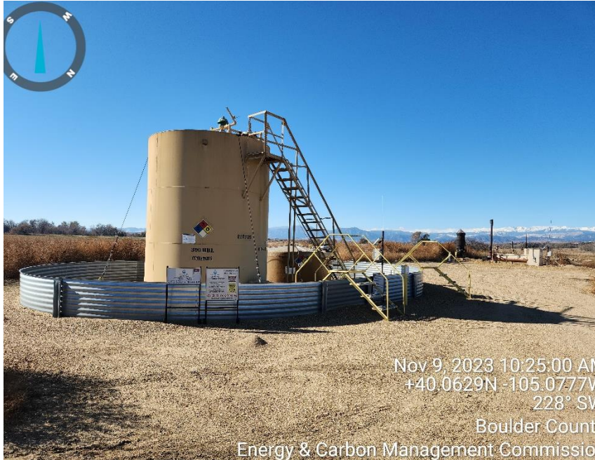
Photo 5 tank battery
