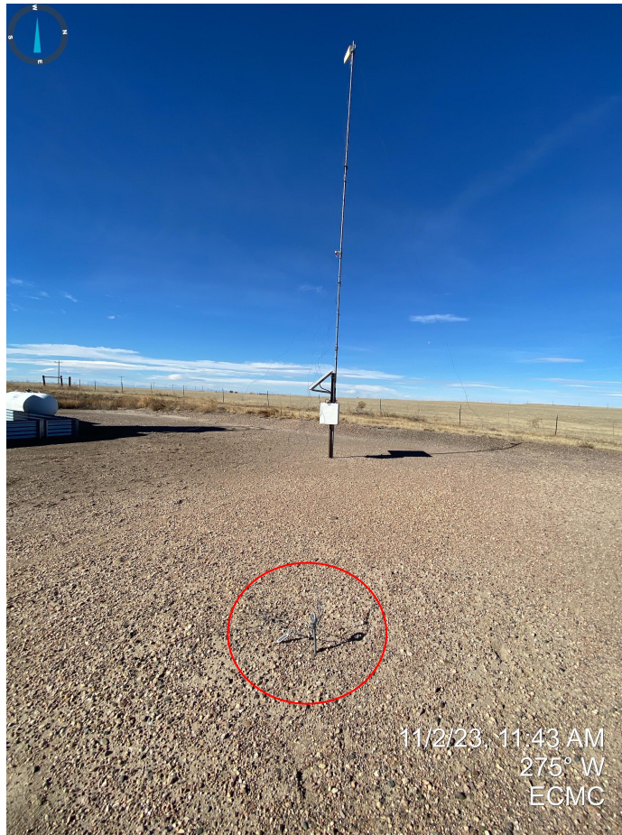
Photo 1. Anchoring equipment (wire) is broken on telemetry equipment.
