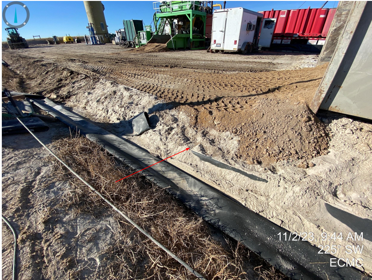
Photo 20. Taken from the eastern side of the location. Photo illustrates unknown and unconsolidated materials within the perimeter stormwater control.
