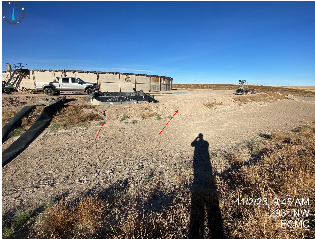
Photo22. Unstabilized soils and erosion degradation (e.g. rilling) occurring within the sediment basin on the northeast corner of the location.
