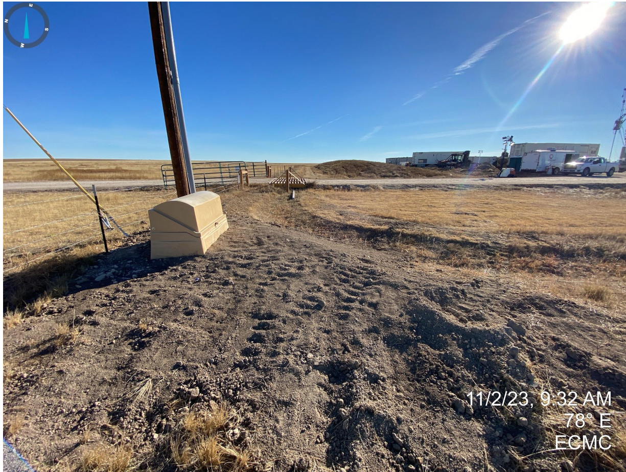
Photo 5. Taken from the northwest corner of the location. Photo illustrates unstabilized soils within the perimeter stormwater control and disturbance area limits. Additional stabilization BMPs are required to prevent erosion degradation from occurring.
