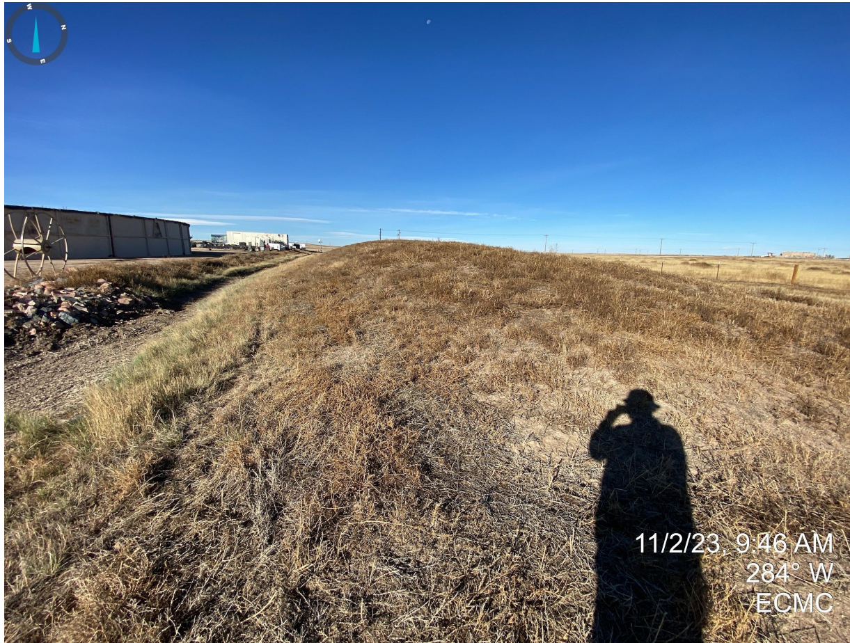
Photo 25. Undesirable vegetation (e.g. kochia and russian thistle) observed on the topsoil stockpile. It appears the weedy vegetation has been previously mowed, however, this is not a substitute for establishing desirable vegetation.
