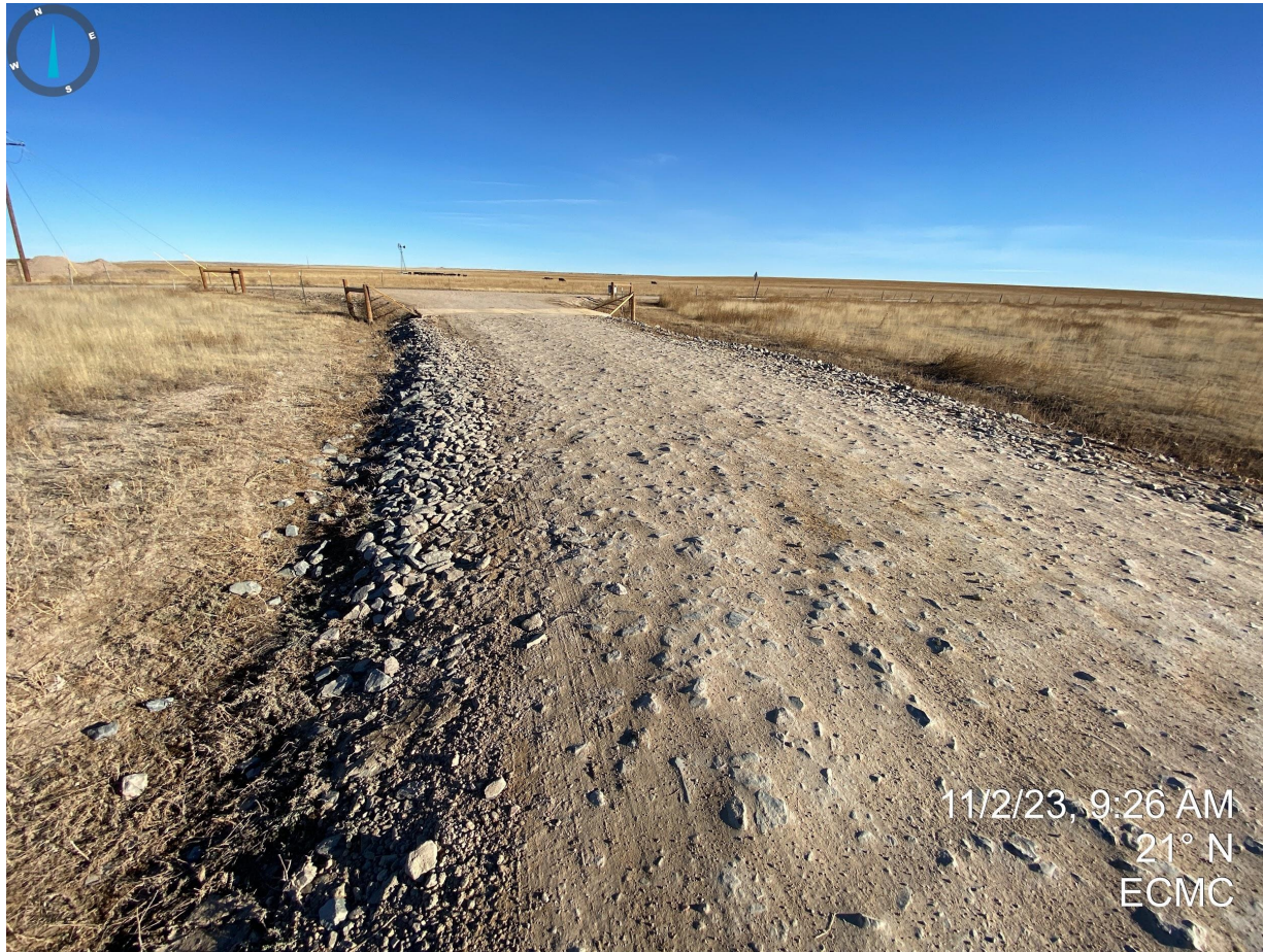
Photo 4. Vehicle track out pad requires maintenance as it is beginning to fill with sediment.
