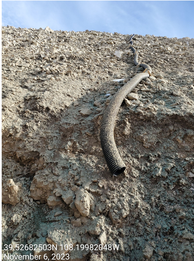
Photo 7: Photo taken from the slope drain on the west end of the Location; outlet protection remains missing per good engineering practices.
