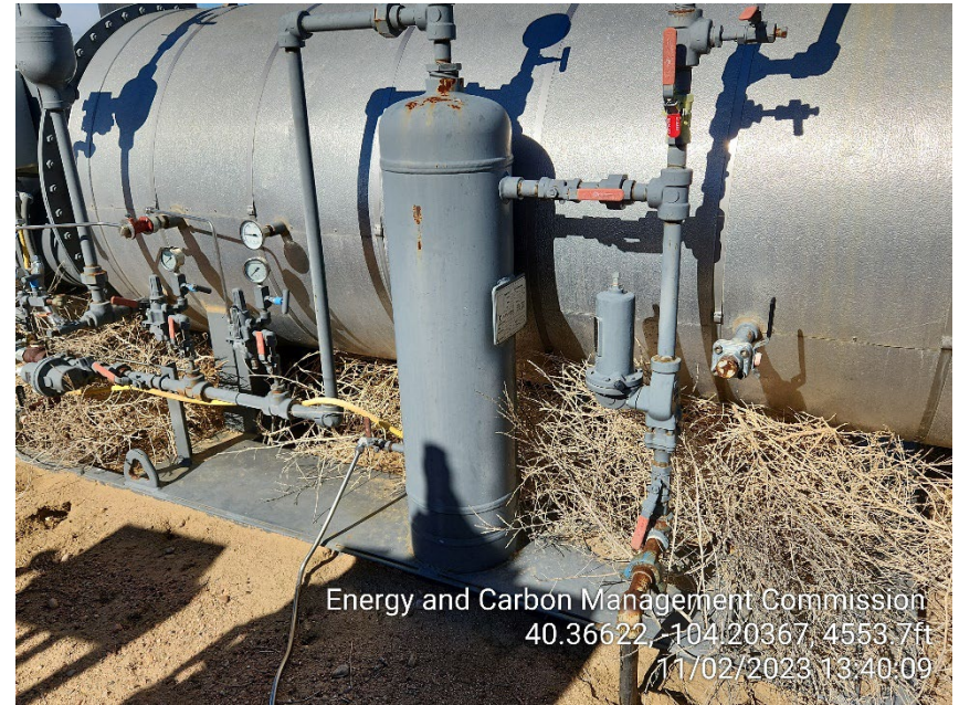
Photo 8 – Line Heater – Tumbleweed Debris
