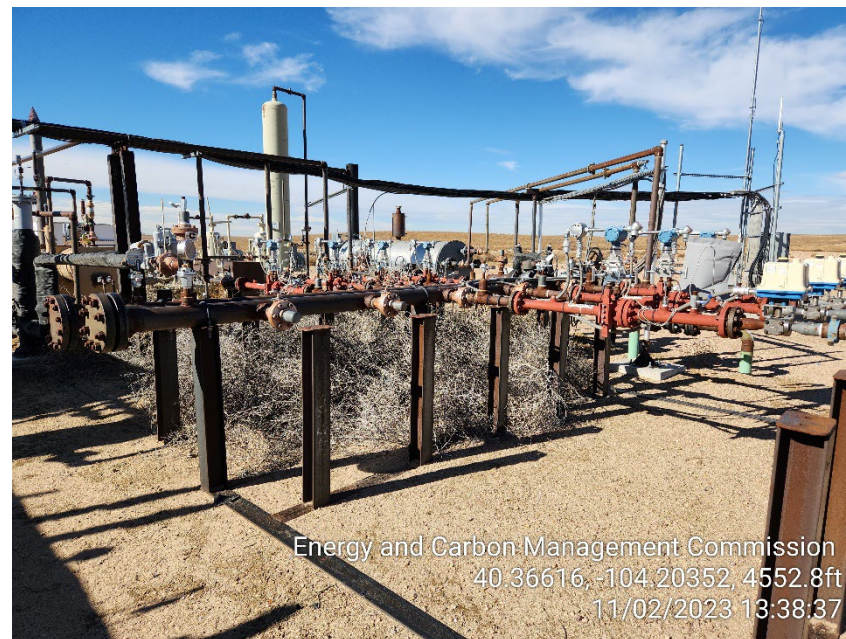
Photo 6 – Gas Meters – Tumbleweed Debris
