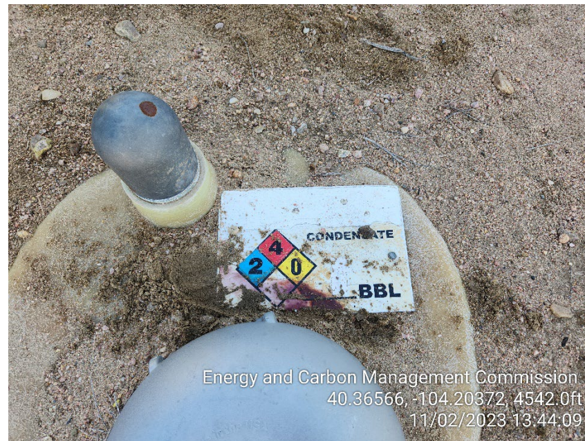
Photo 14 – Capacity Label missing – NW Corner on Tank Berm
