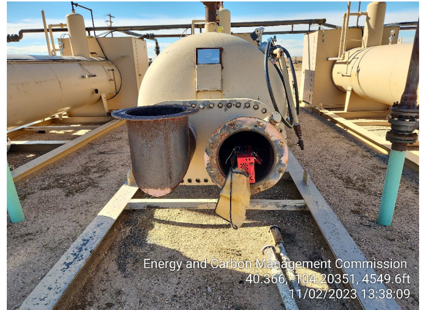
Photo 4 – South Separator – Open
