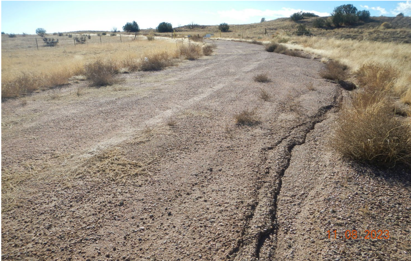
Photo 1. Facing southeast at the beginning of the access road. There is erosion occurring along the road.
