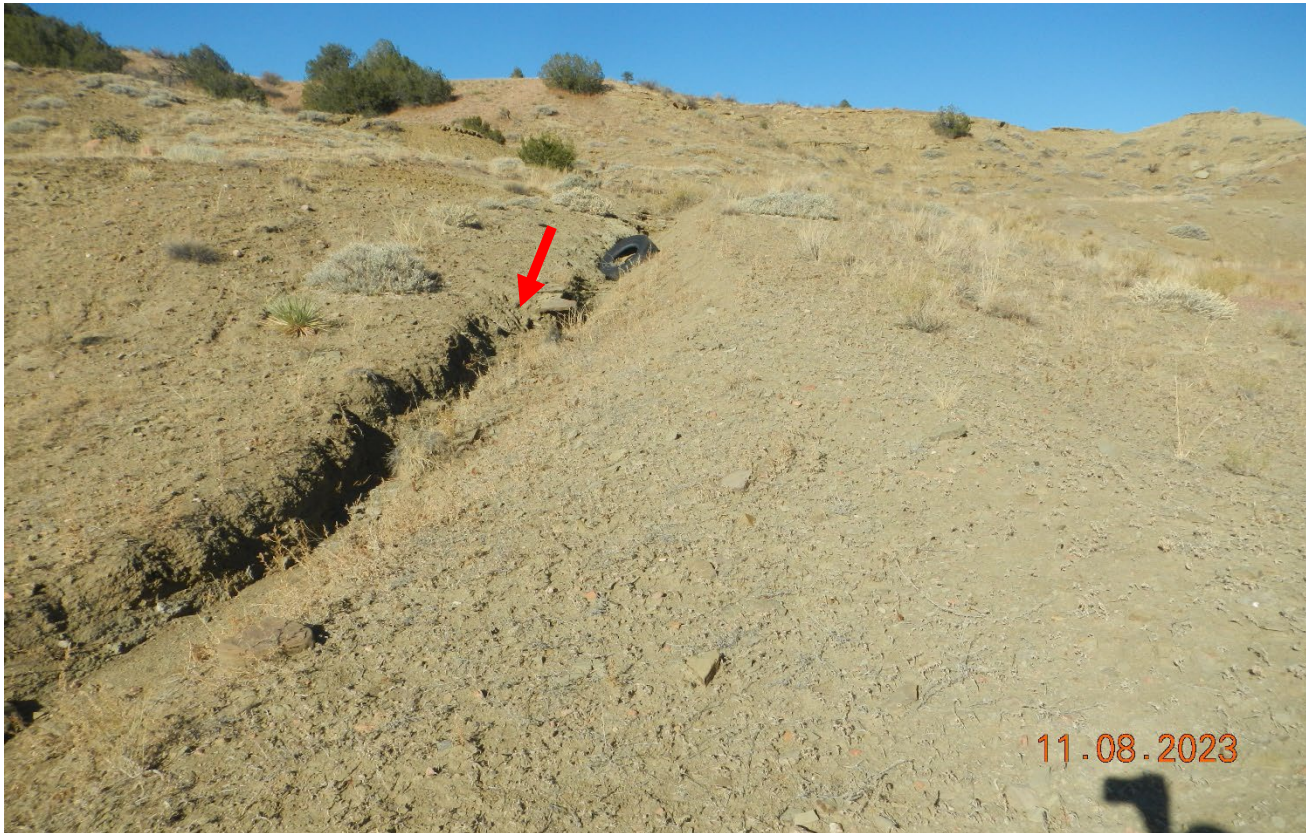
Photo 7. Facing west at the south side of the location. There is an erosion channel shown at red arrow which will need to be repaired and stabilized.
