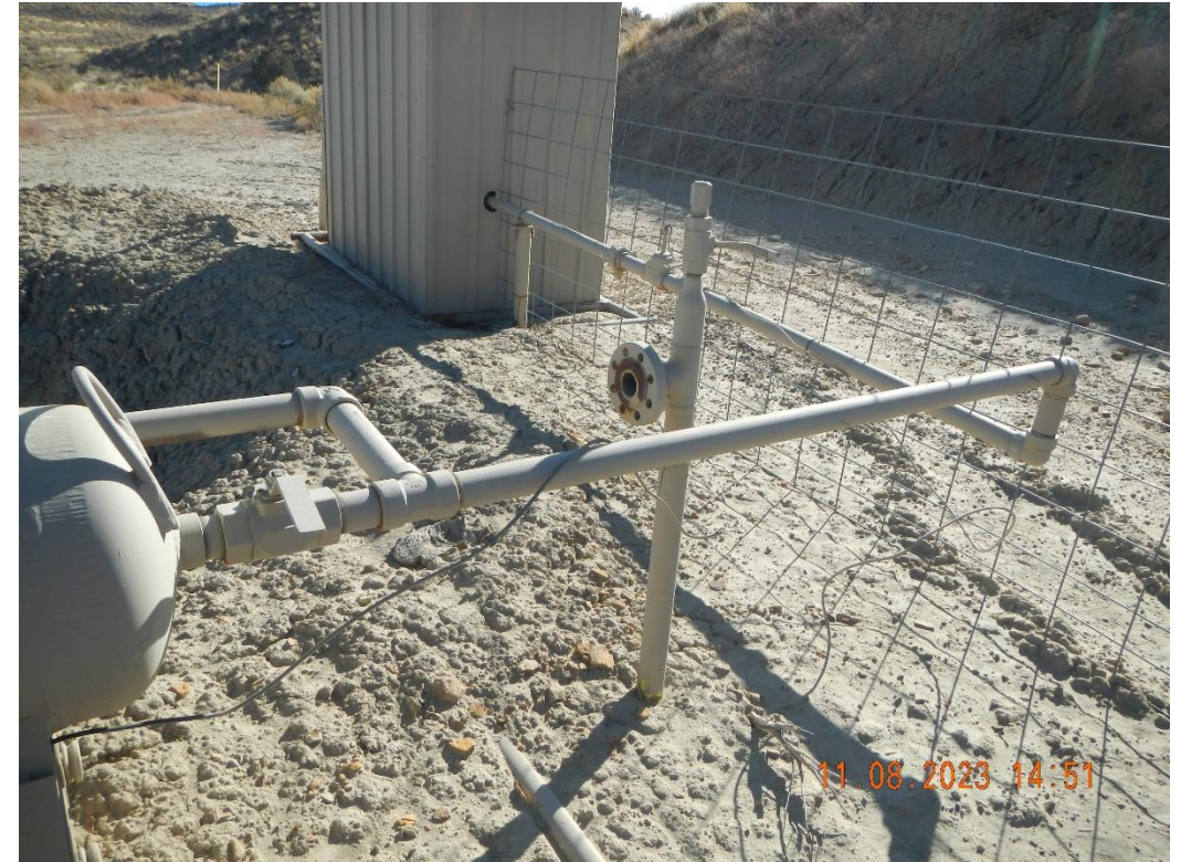
Unused 2" riser at pit and surface equipment. No OOSLAT
