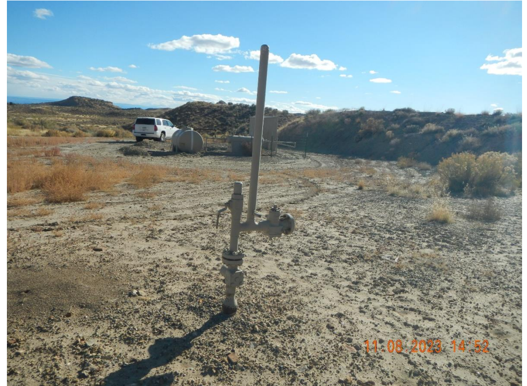
1-UGC riser just north of the pit and surface equipment.
