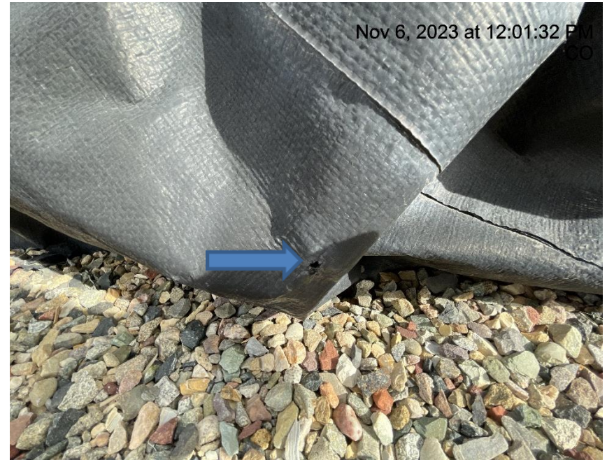
Photo # 5553 Hole in liner/liner needs maintenance
