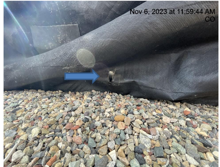
Photo # 5551 Hole in liner/liner needs maintenance
