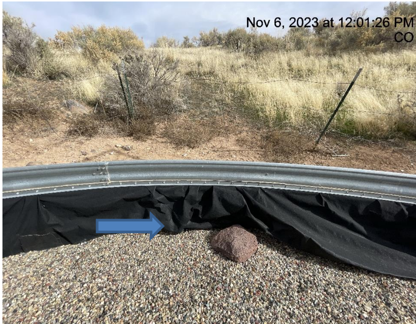
Photo # 5552 Hole in liner/liner needs maintenance
