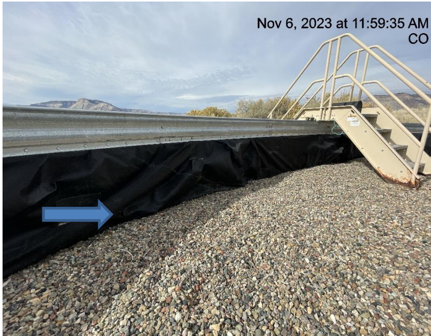
Photo # 5550 Hole in liner/liner needs maintenance
