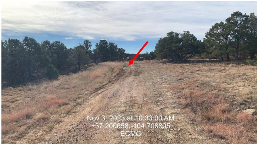
**Photo 7 – Main Access, Vehicle Rutting**
