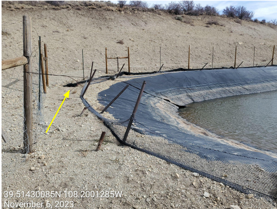
Photo 5: Photos show netting (arrow) has not been replaced over the pit.
