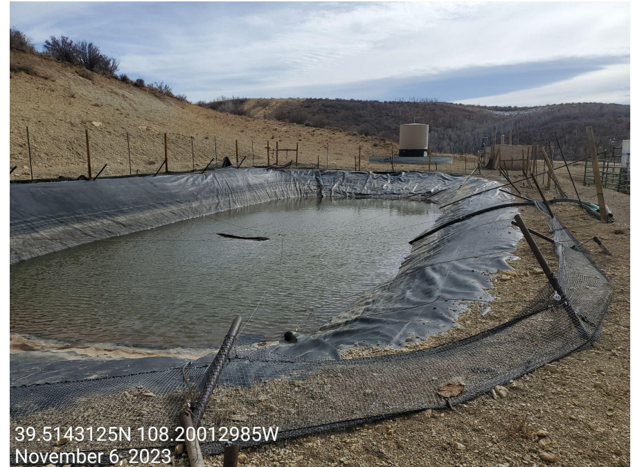
Photo 5: Photos show netting (arrow) has not been replaced over the pit.
