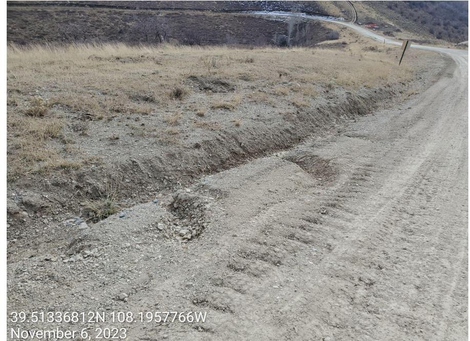
**Photo 7:** Photos taken from the access road. Previous inspection observed that stormwater runoff from the Location has resulted in degradation the Location's entrance and access road. The Location entrance has been re-constructed, however erosion degradation along the access road remains apparent.
