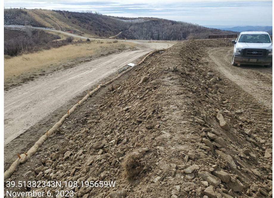
**Photo 3:** Photos examples showing berm constructed along the perimeter of the WPS; erosion logs implemented along the Locations disturbance.
