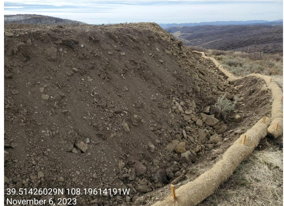
**Photo 4:** Photos examples showing slopes of the Location are bare, lack stabilization and are at risk to wind and water erosion; stormwater and erosion control measures inadequate.
