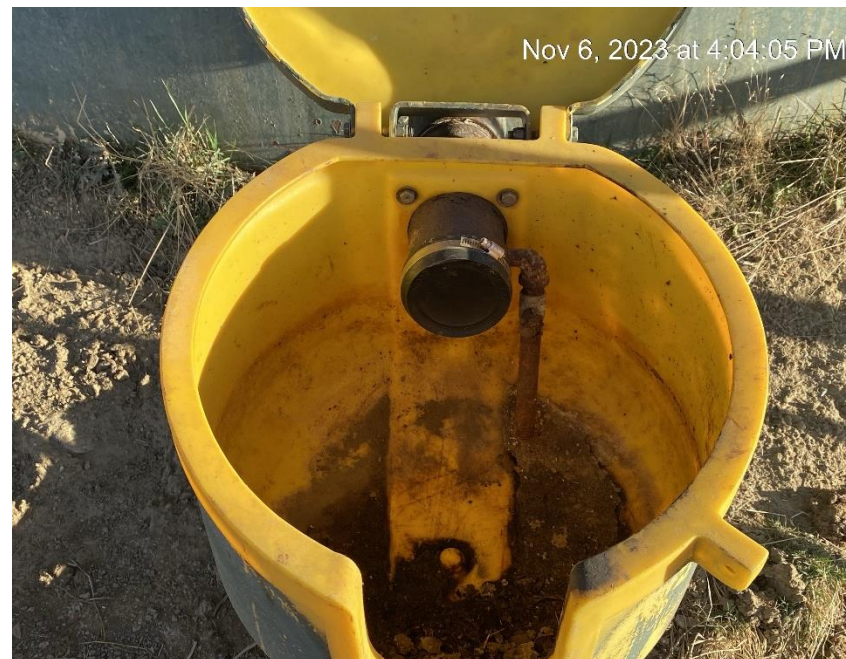
Insufficient cap on loadline
