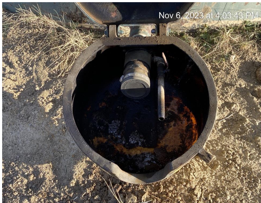
Insufficient cap on loadline
