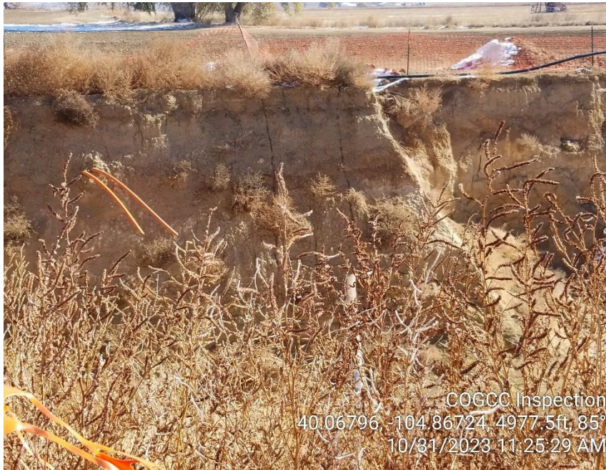
Photo 7 – Exposed flowlines in open excavation.
