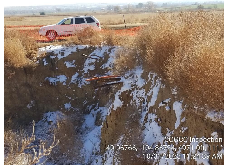
Photo 8 – Exposed flowlines in open excavation.
