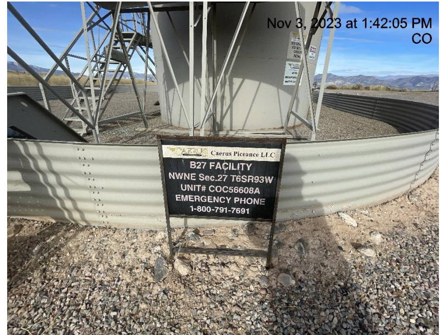
Photo # 5405 Battery sign lacks required info
