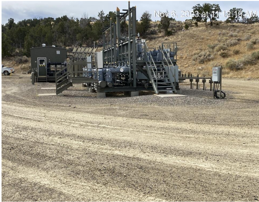
Facility from Northeast corner
