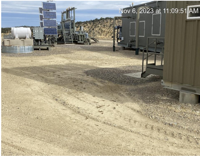
Facility from Southwest corner
