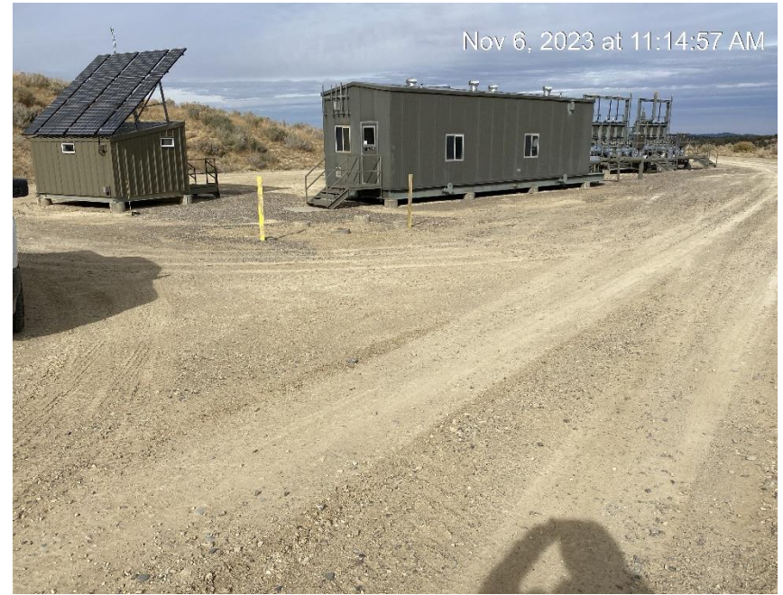
Facility from Southeast corner
