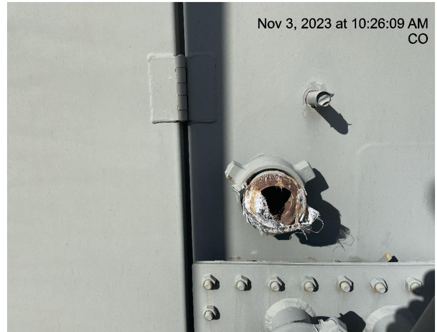
Photo # 5219 Open ended pipe on production separator/ wildlife hazard
