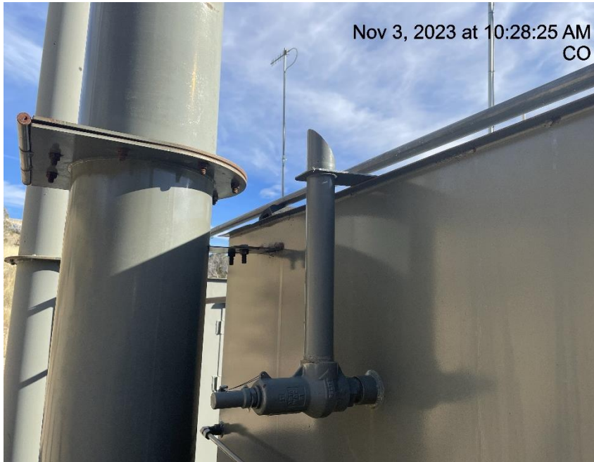
Photo # 5224 PRV vent line lacks cap
