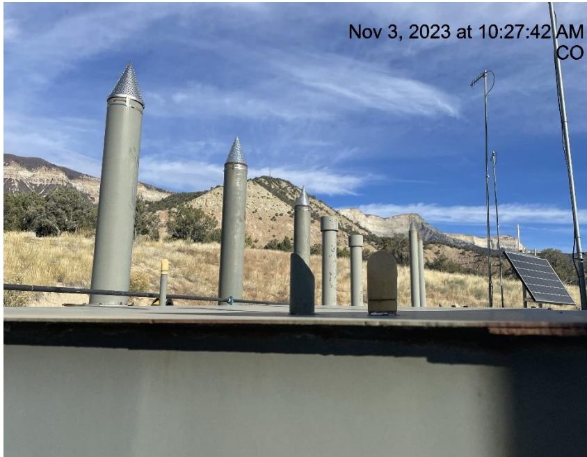
Photo # 5222 PRV vent line lacks cap
