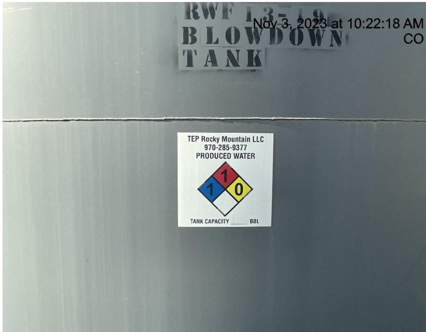
Photo # 5230 Capacity on tank label on blowdown tank faded & illegible
