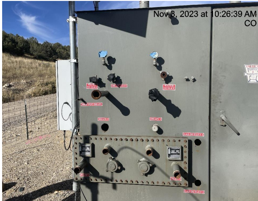
Photo # 5216 Open ended pipes on production separators/ wildlife hazard
