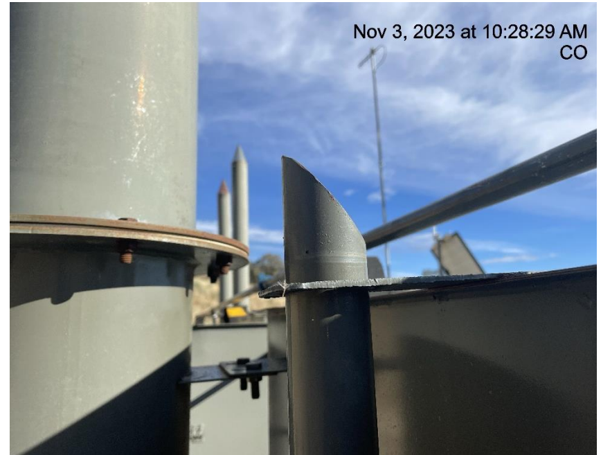
Photo # 5225 PRV vent line lacks cap
