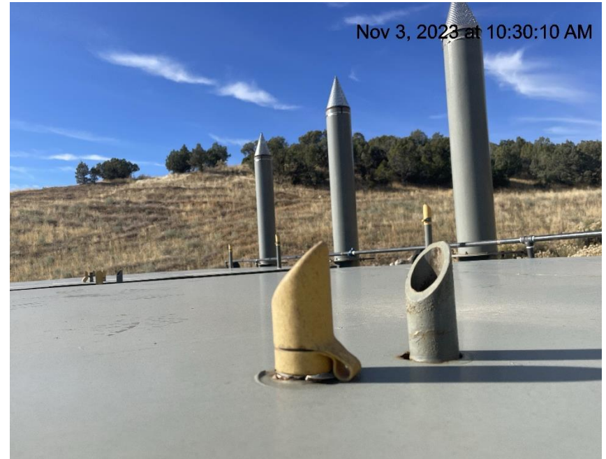
Photo # 5227 PRV vent line lacks cap
