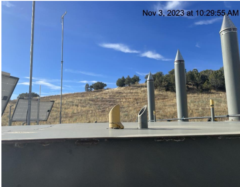
Photo # 5226 PRV vent line lacks cap
