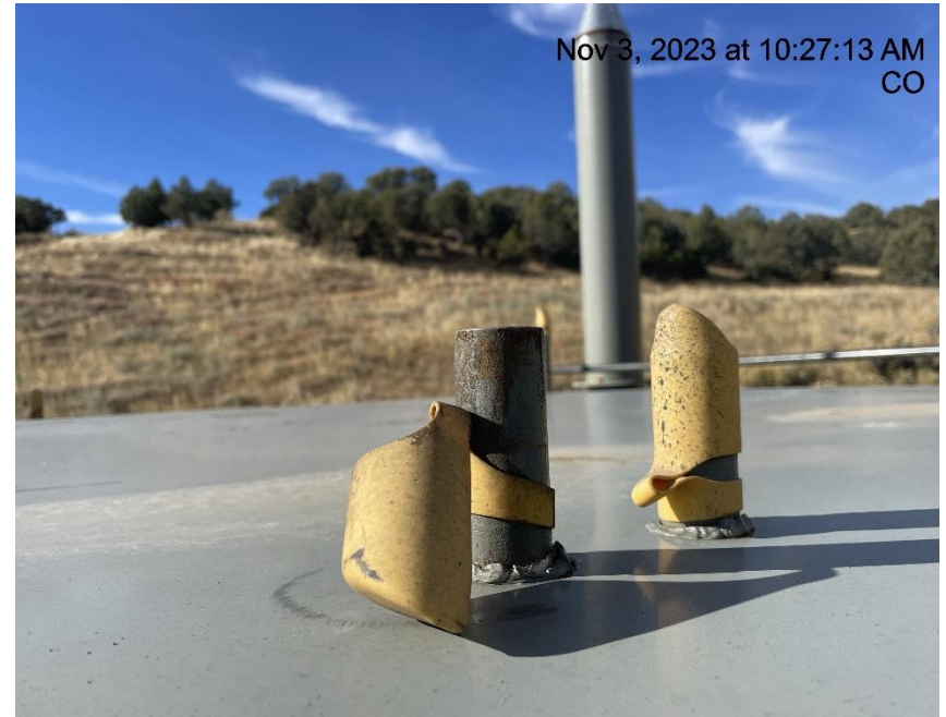
Photo # 5221 Rupture disc vent line not capped
