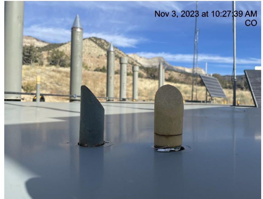
Photo # 5223 PRV vent line lacks cap
