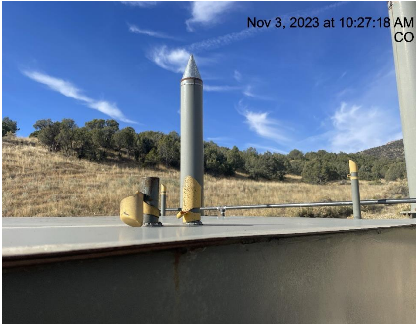
Photo # 5220 Rupture disc vent line not capped
