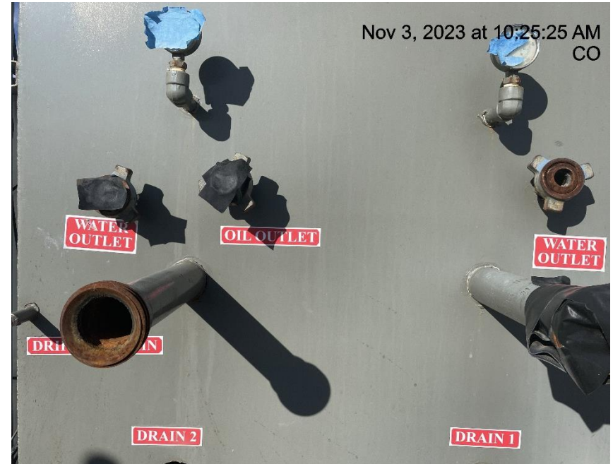
Photo # 5217 Open ended pipes on production separators/ wildlife hazard
