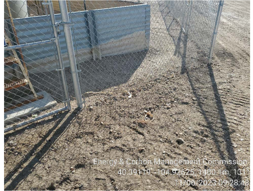
Erosion BMP's on 11/6/2023
