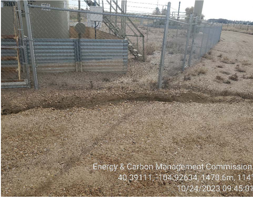
Erosion BMP's on 10/24/2023
