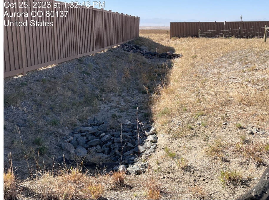
Photo 4. Photo taken of drainage ditch around pad, with large rock check dams and rock rundowns to culvert. Photo taken facing west.
