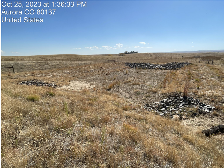
Photo 9. Photo taken of sediment basin and rock check dams in drainage leading to it. Photo taken facing southeast.
