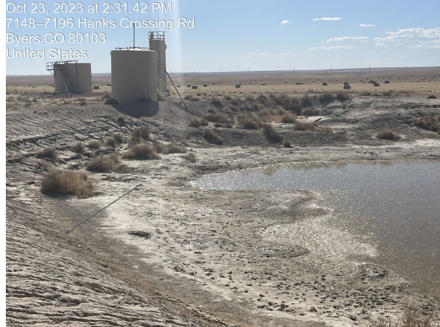
Photo 8. Photo of weeds (Kosha & russian thistle) around produced water pit and reeling on pit walls facing southwest. Pit # 107681
