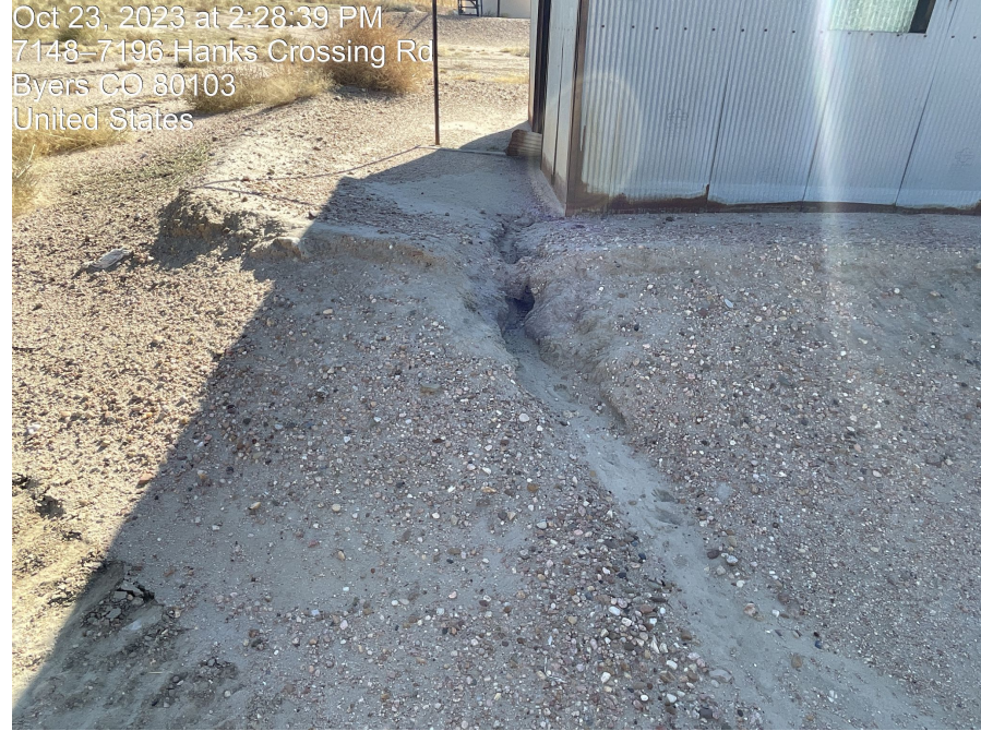
Photo 6. Photo of breached berm around equipment on site facing north.
