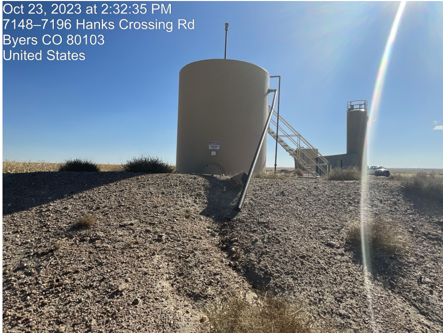
Photo 9. Photo of produced water tank emptying into pit on site, facing south
